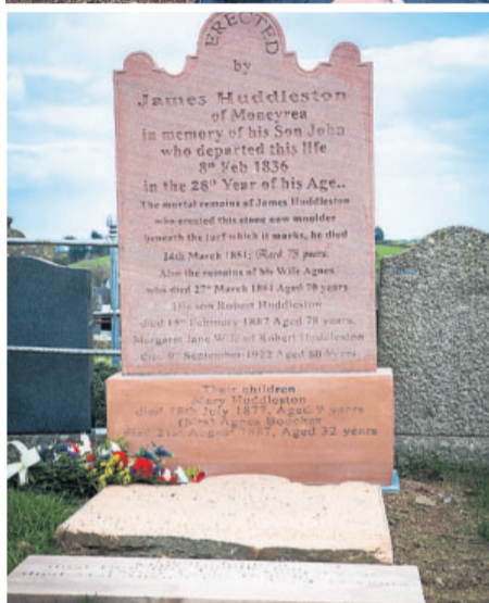
The replacement headstone to the Huddleston Family in Moneyreagh Churchyard, with the original broken headstone covering the grave
